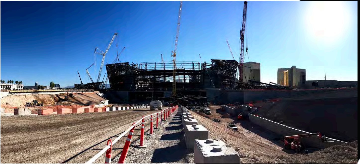
Above: Panorama view from the temporary ramp looking north.
